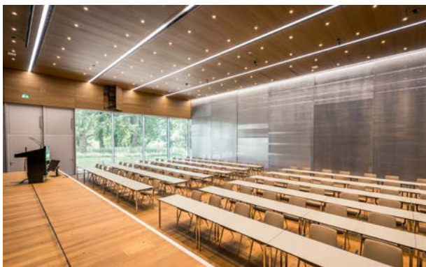
Dividing Wall: The hall may be divided by means of an acoustically transparent metal curtain. This is ideal for a smaller number of people.
